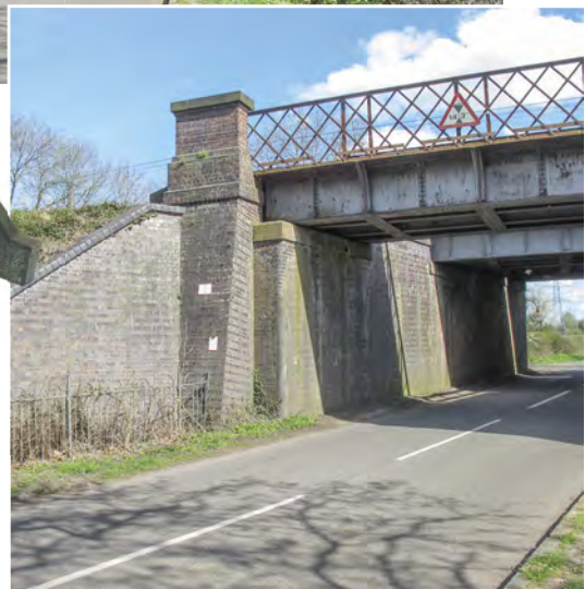
Looking at the prototype, you can see how the girders and parapet tuck inside the pilasters. Modellers tend to try and stretch the model by fitting them on the inner ends but this would be too flimsy in real life.
