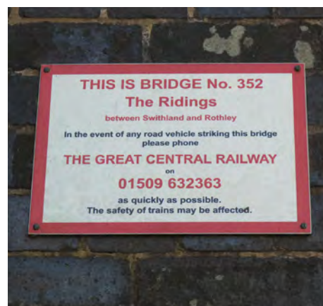
Bridge sign – Don't forget if a road passes under your bridge, you need to fit a sign to the parapet to let lorry drivers know if they can squeeze underneath.
