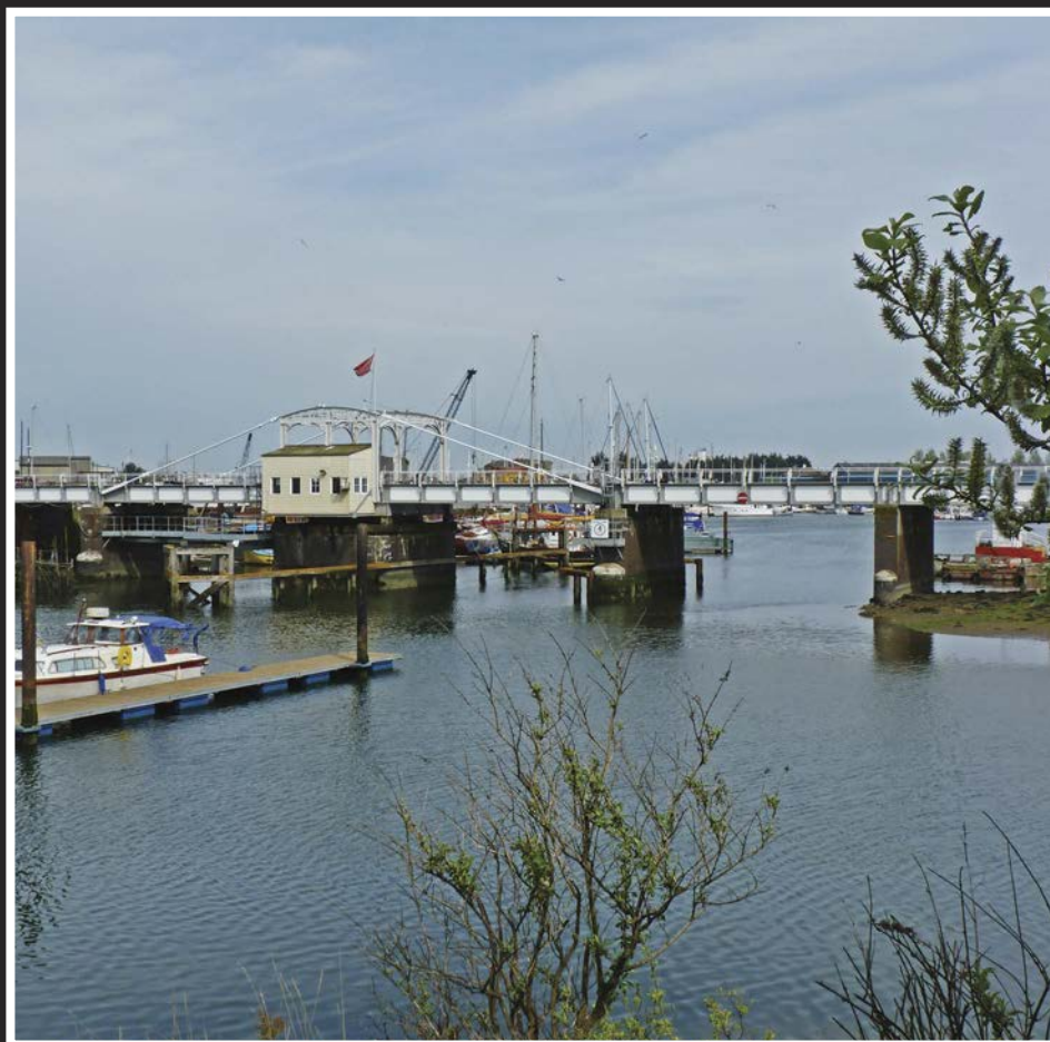
Crossing Oulton Broad, this swing bridge has carried the Lowestoft-Beccles line since 1905. Its original electrical and mechanical operating systems are currently being upgraded by Network Rail to give greater safety and reliability. Note the fenders preventing vessels colliding with the bridge piers.
