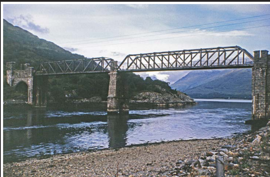
Creagan Bridge in 1984. Opened as part of the Callander & Oban Railway, Ballachullish branch line, in 1901, the steel, lattice trusses mounted on granite towers stand idle following the closure of the line in 1966. A new lease of life awaits!
