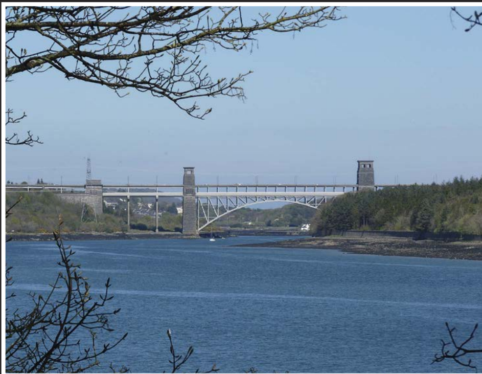
Britannia Bridge, once a tubular type, links the mainland with the Isle of Anglesey. The masonry tower to the right of this image is the centre support and larger than its two outer counterparts; a second steel arch is to its right. Road traffic takes the upper deck, added in 1980.
