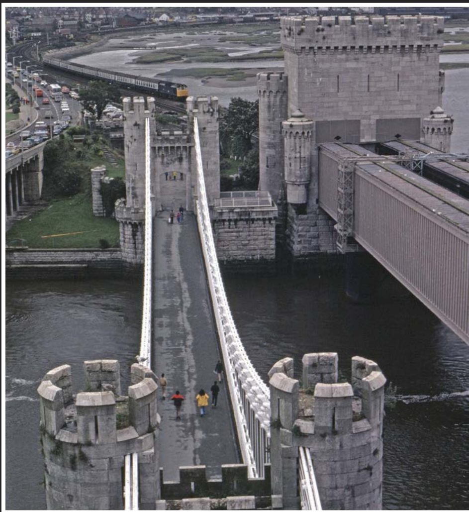
Conwy railway bridge is to the right of this image. The older suspension bridge in the centre once conveyed the Chester-Bangor road before being replaced in 1958. The Class 25 locomotive is about to head its train through the right-hand portal of the castellated tower and pass through the up-line tube of the railway bridge, en route for Llandudno Junction. Note the supporting piers emerging from the river bank.
