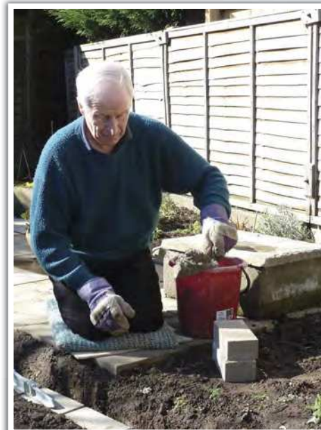
Carefully laying blocks with the aid of a spirit level.
