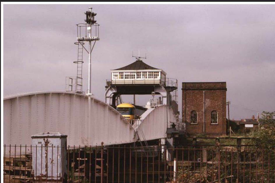
Prior to the 1983 re-routing of the East Coast Main Line, a Class 43, HST passes beneath the control cabin, while traversing the movable span of Selby swing bridge. To the right is the brick building that housed the accumulator supplying hydraulic power to the engines that turned the bridge. Note the light standard mounted on the nearest span controlling river traffic.
