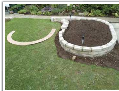
Cheap plywood templates showed me where to dig my trenches.
