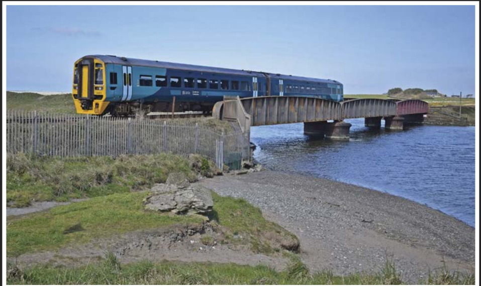
Crossing the 'Broad Water' on the Cambrian Coast Line to the north of Tywyn is this single-track bridge; consisting of three spans of hogback steel girders, it replaced the original timber bridge in 1911.
