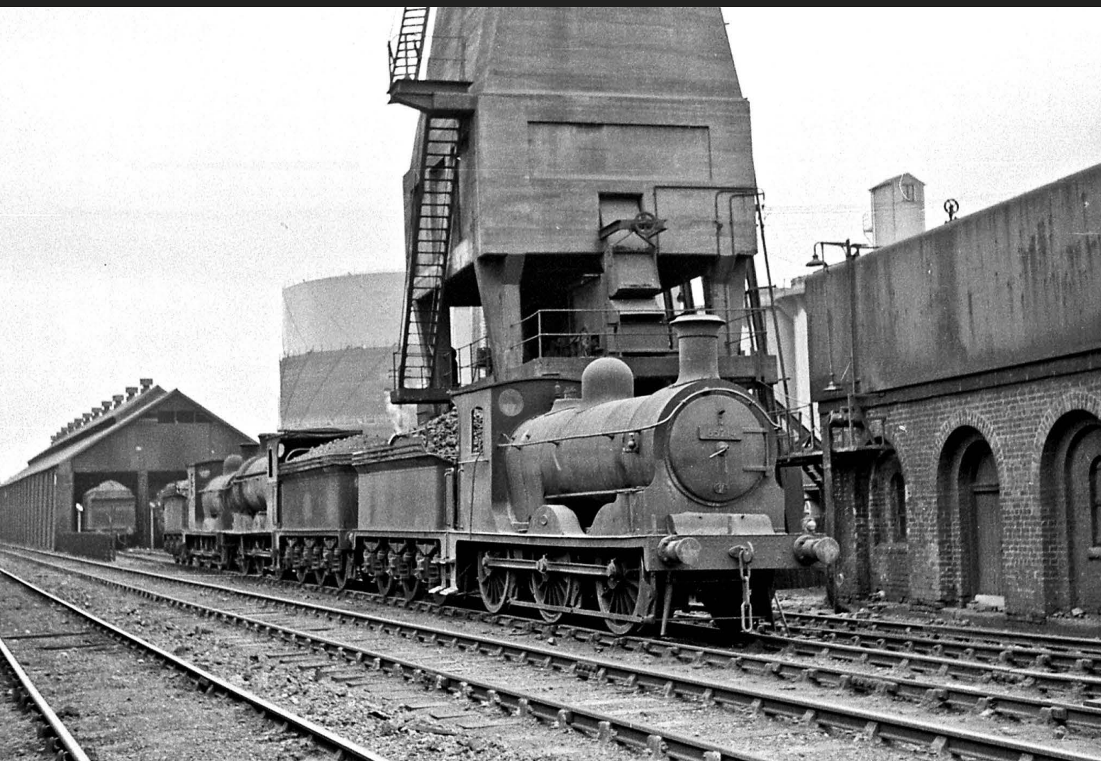
BELOW: No. 65214 is at the head of a line of classmates captured alongside the coaling tower at Kipps depot, near Airdrie. Note how many of the frames and cab footsteps on these locomotives appear to droop, no doubt due to the occasional rough shunt over their many years of service. A hose can be seen exiting the cabside window.
