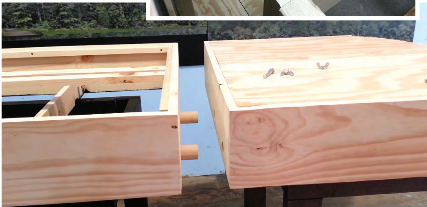
Large wooden dowels were used to align the modules and keep them tightly together.
