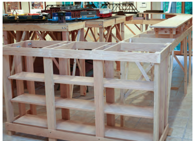
This view of benchwork in its early stages of construction shows how I incorporated storage shelves as part of the framework.
