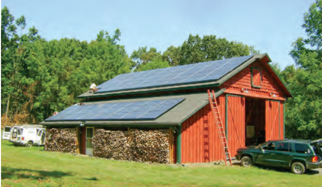
Solar collector panels were mounted on the roof of a structure on the RMT headquarters property. The RMT system is rated at approximately 16 kilowatts and required 68 panels of 245 watts each interconnected into six strings of panels.
