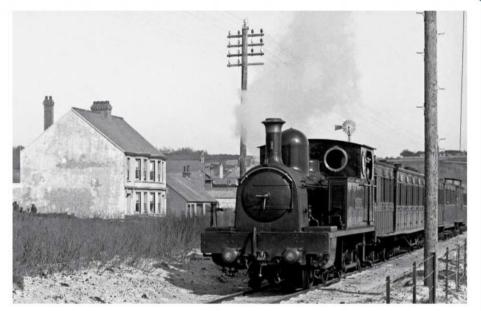
The rebuilt 3ft 6in gauge Jersey Railway started with two 1884-built Manning Wardle 2-4-OTs, Nos. 1 St Heliers and 2 St Aubyns. No. 1 is photographed on the sea-front section between St Helier and St Aubyn - part of this stretch was built on a wooden viaduct before the sea front was extended onto land reclaimed from the sea. RAIL ARCHIVE STEPHENSON
