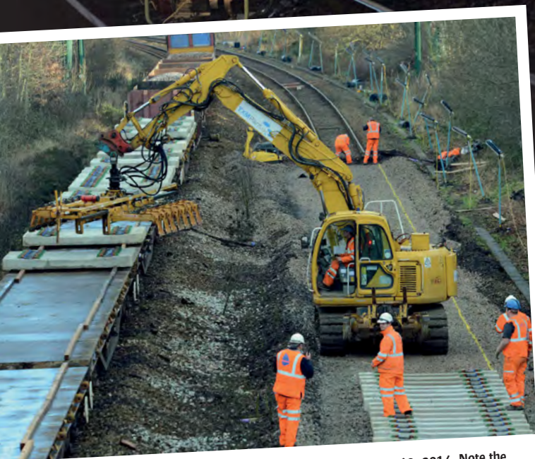
The 'Up Main' at Mytholmroyd undergoes track renewal on January 19, 2014. Note the panel grab particularly useful for unloading several sleepers at a time from wagons.
