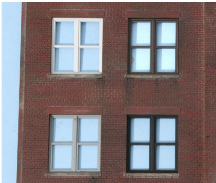
Fig. 7 Hiding oversized parts. Due to limitations in injection-molding technology, parts are often cast oversized. By painting these parts a dark color, you can downplay the problem.
