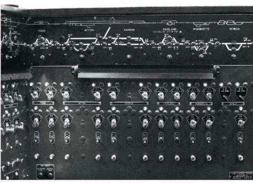
The most efficient way to move a lot of trains is Centralized Traffic Control, represented here by a Union Switch & Signal CTC "machine" at Springfield, Mo., on the old St. Louis-San Francisco. A machine like this also makes a great toy for a model railroader. Harold A. Edmonson photo
