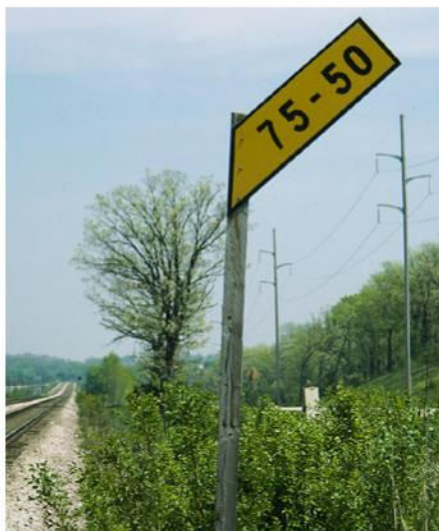
This former Milwaukee Road speed sign has limits for both passenger and freight trains. Robert S. McGonigal photo
