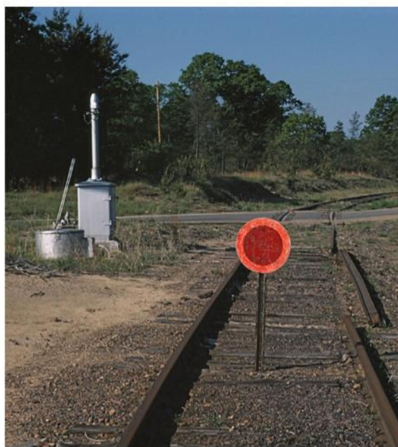
Red boards, placed either next to track or between the rails, mean stop. Gordon Odegard photo
