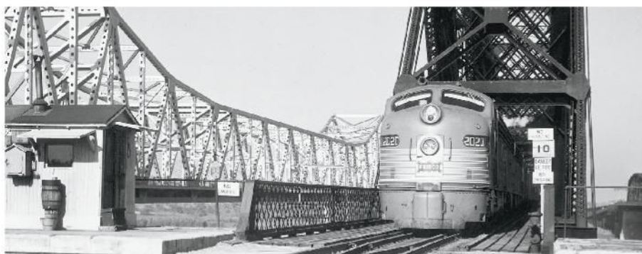
Bridge approaches often feature a collection of warning signs, as at the St. Louis-San Francisco's Mississippi River bridge at Memphis, Tenn. The bridge has a 10 mph speed limit. James G. La Vake photo
