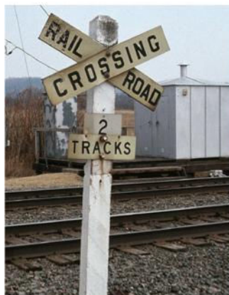
This ex-Chicago, Burlington & Quincy crossbuck has sharply angled signboards. You can still see the pattern for the zebra stripes once painted on the concrete post. Jeff Wilson photo
