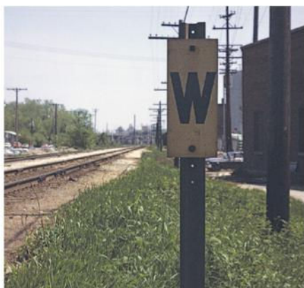
Typical of more-modern signs along the right-of-way, this Milwaukee Road whistle marker has a metal signboard mounted on a formed steel post. Gordon Odegard photo
