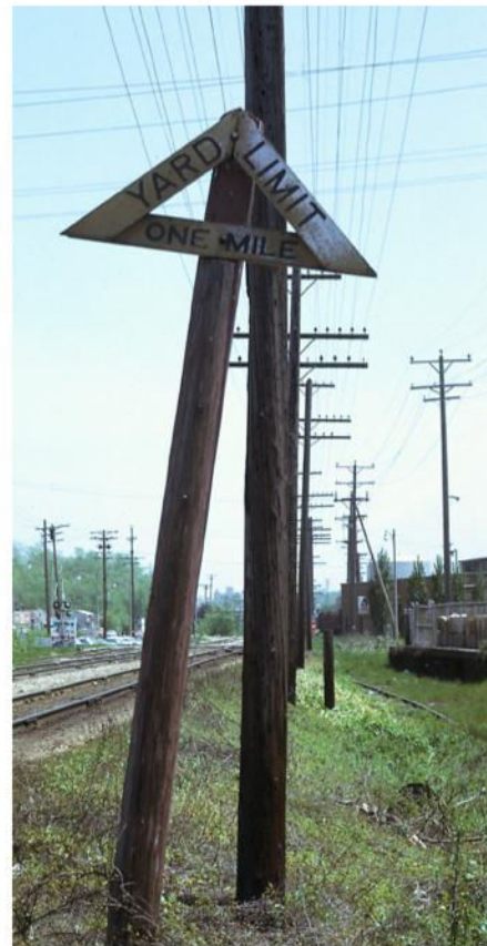
This sign, a mile away from a yard limit board, warns engineers to approach the yard limit with their trains under control. Gordon Odegard photo
