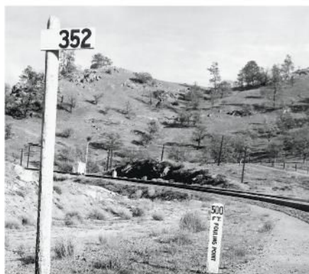
This small sign to the right of the milepost marks the distance to the fouling point of a junction switch.
