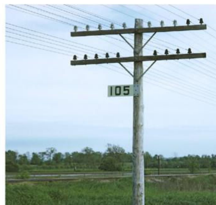
Since line poles were already in place along their rights-of-way, some railroads simply had them do double duty by attaching mile markers to them. Gordon Odegard photo
