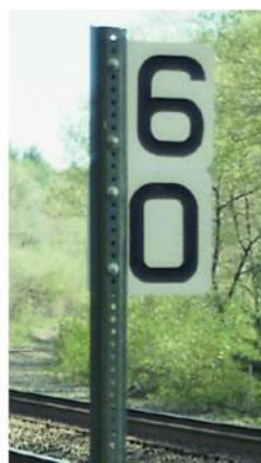
Modern mileposts usually have sheet-metal signs bolted to steel posts. Jeff Wilson photo
