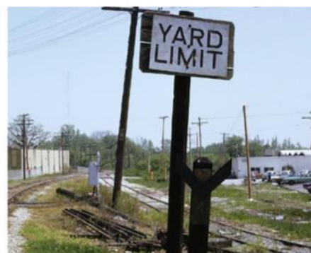
Just in front of and below the yard limit sign stands a V-shaped flanger post. Gordon Odegard photo
